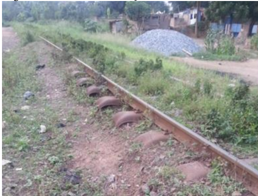
Figure 2-10: A section of tracks with weeds
